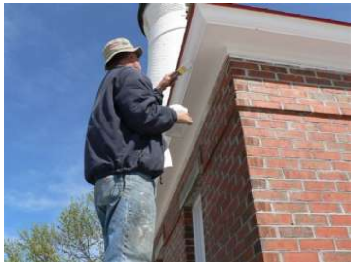
Rick painting the trim outside the service building.
