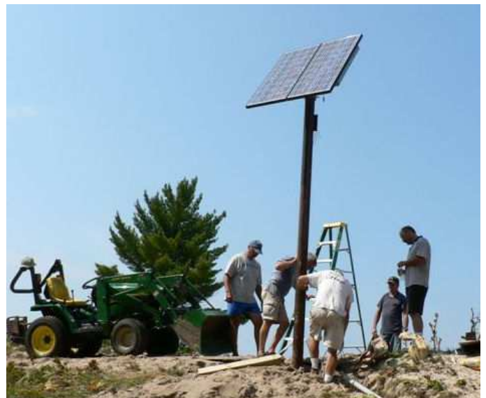
Installing the solar system
